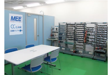
Conformance testing lab
